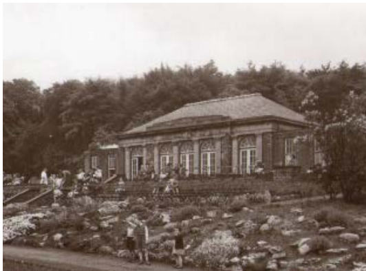
Pavilion building circa 1930's
