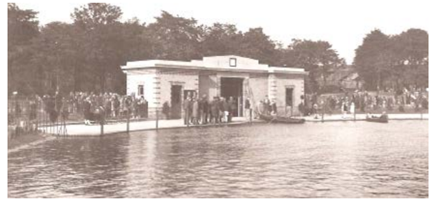
Boat House as constructed
